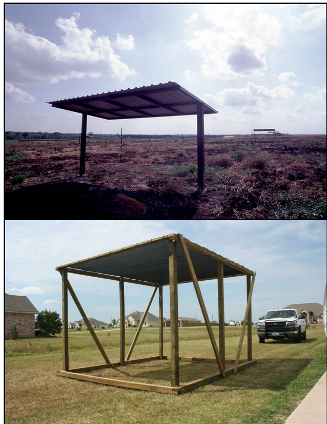
Figure 16. Shade structures constructed with a tin roof (top) and a shade cloth (bottom). Photos courtesy of The Samuel Roberts Nobel Foundation Inc. (top) and Larry Redmon, Texas AgriLife Extension Service.
