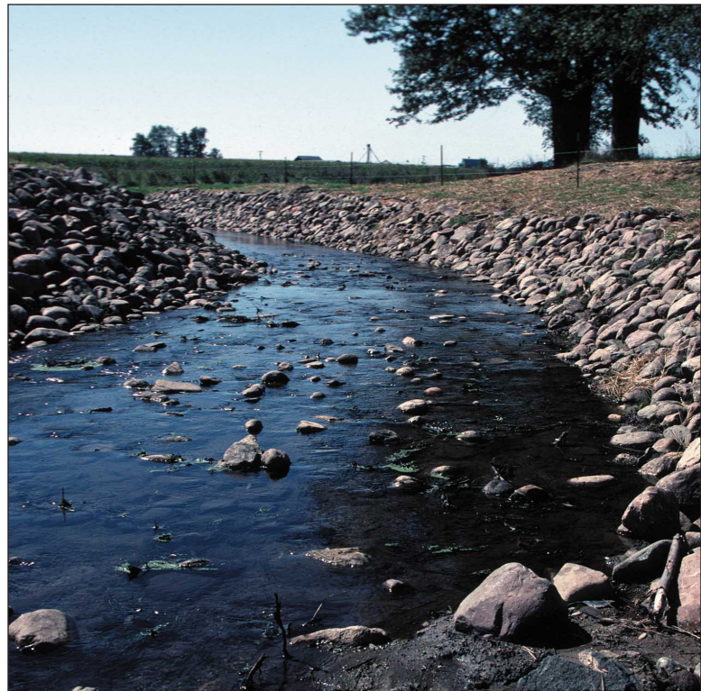
Figure 20. This stream bank has been stabilized from erosion with rip-rap. Photo courtesy of the USDA-NRCS.
