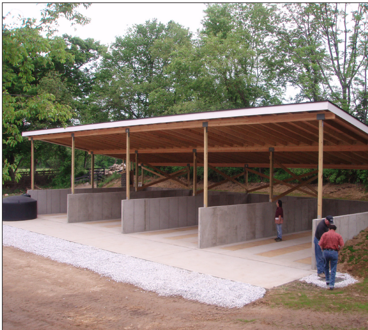
Figure 24. Multiple bin horse compost system. Photo courtesy of O 2 Compost.
