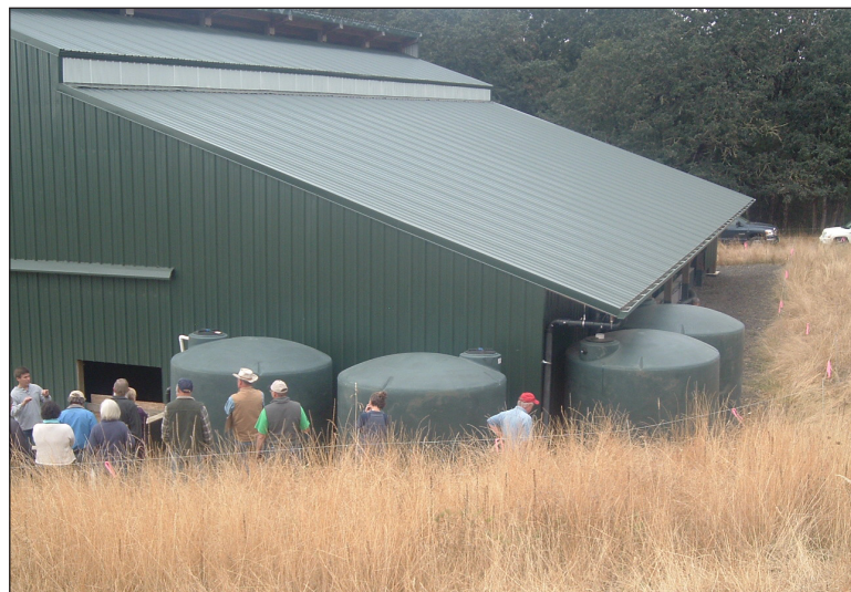
Figure 15. These four 2,500-gallon water harvesting tanks capture rainwater from the barn’s roof and help save more than 162,000 gallons of water a year that would otherwise be pumped from the groundwater aquifer. Photo courtesy of Yamhill Soil and Water Conservation District.
