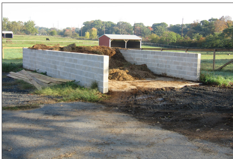
Figure 21. Dry stack horse manure storage area. Photo courtesy of the Livestock and Poultry Environmental Learning Center.
